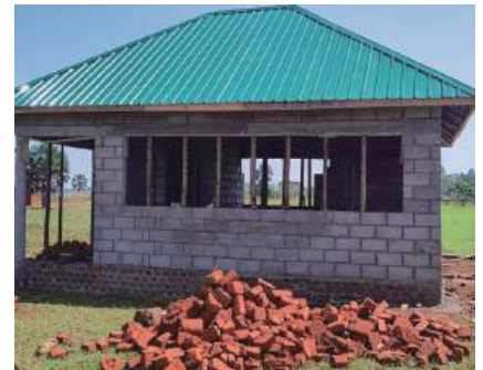
Kitchen under construction
